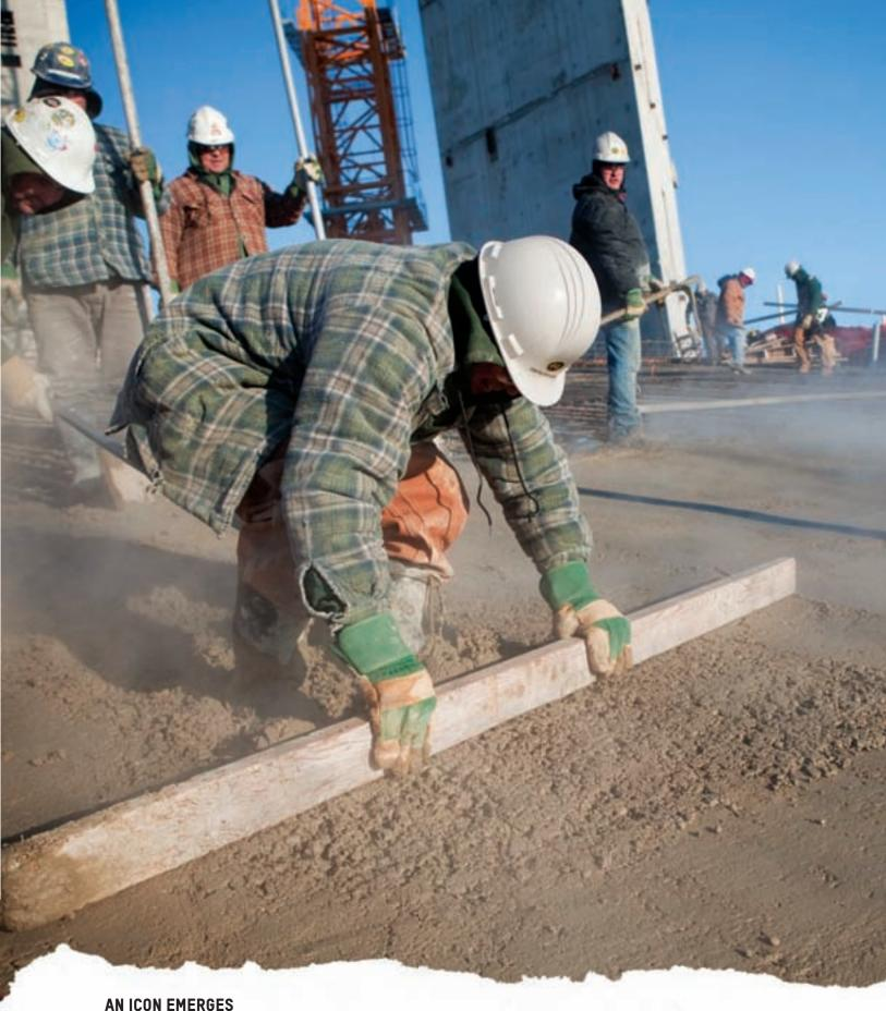
Construction crews work on the Museum's concrete foundation. To put the Museum's size into perspective, if all the concrete used in the Museum were brought to the construction site at one time it would take 2,125 fully loaded cement trucks to deliver it. The building's skeleton has the same amount of steel as 27 diesel-electric locomotives, and the Museum's floor plan will be equal in size to four CFL football fields combined.
